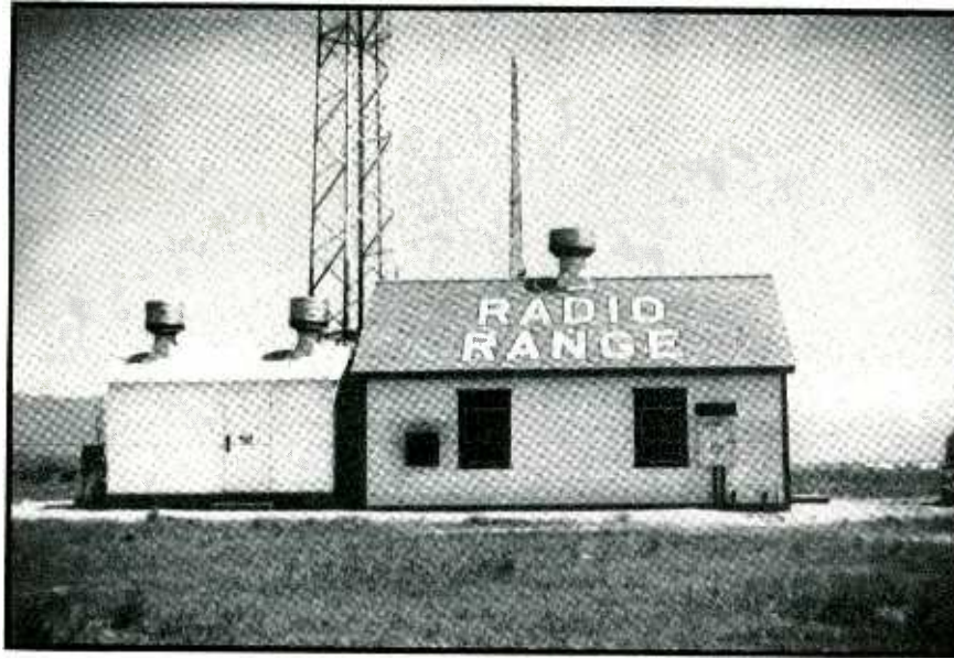
CLOSE-UP OF THE FIVE-TOWER RADIO RANGE STATION.
