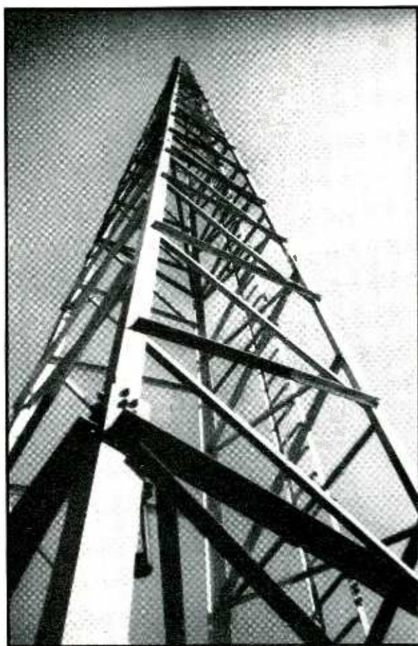
One of the 120-foot vertical towers forming a part of the radio range station.
